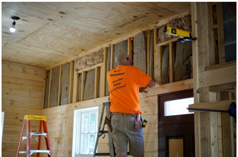
Top: Jim Seville paints the window trim on a window on the west wall of the Roundhouse. – Al Gallo photo
