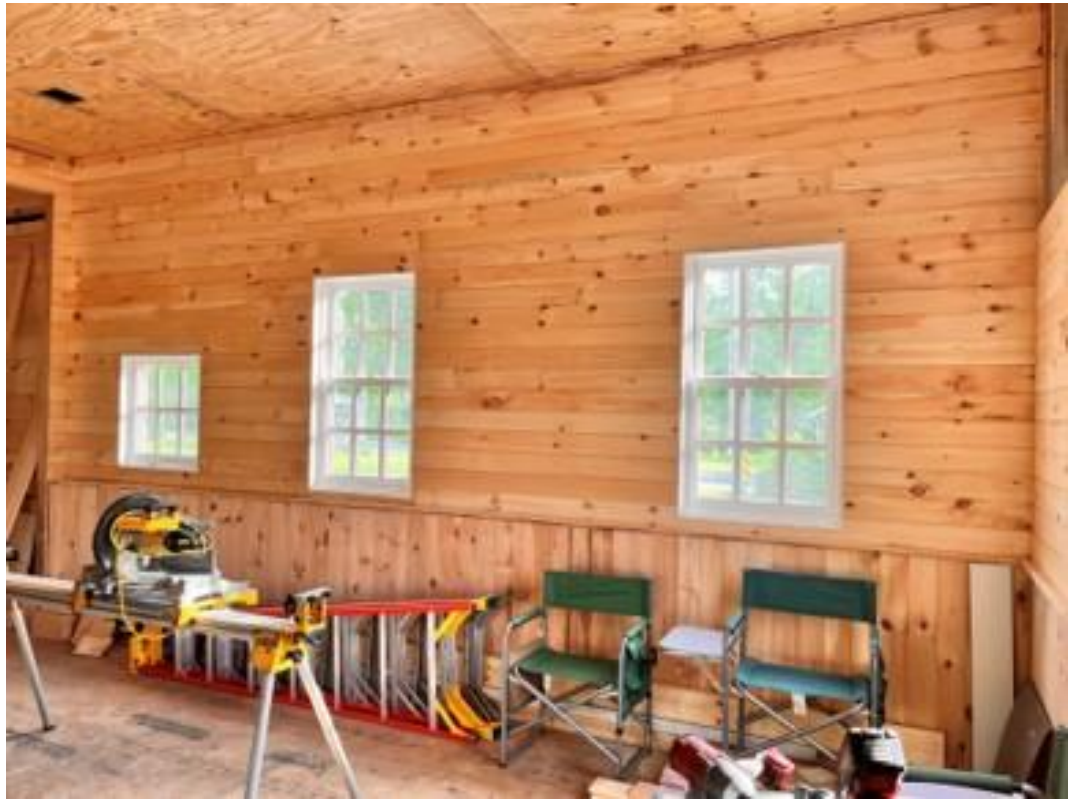
Above: Siding work in the Saltillo Station waiting room is nearing completion. – Dave Bulman photo
