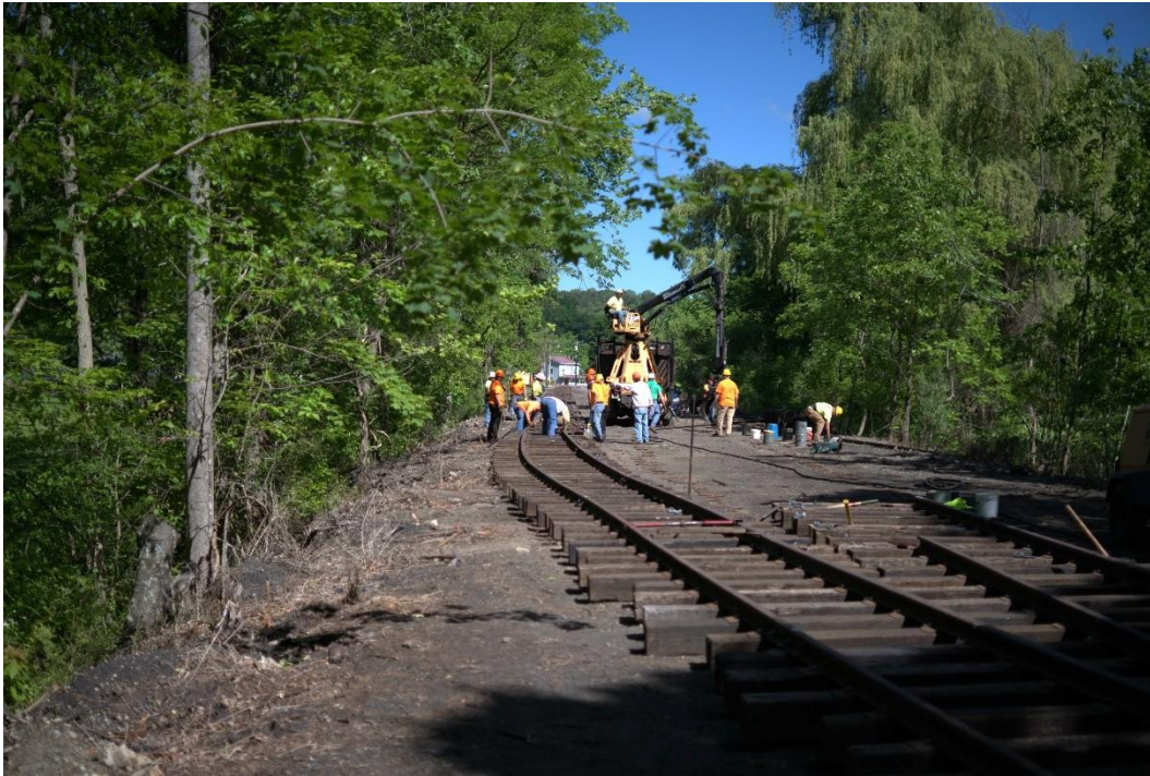
The EBTF/FEBT Track Crews connect the Saltillo station siding to the newly built north switch in the main line during the Spring Work Week. – Al Gallo photo
