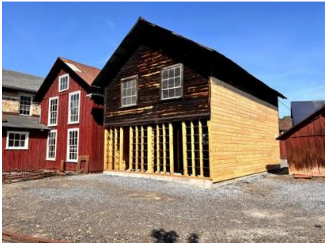
Below: New center posts, completed stock racks, and new replica siding have been installed on Storehouse 2. – Dave Bulman photo
