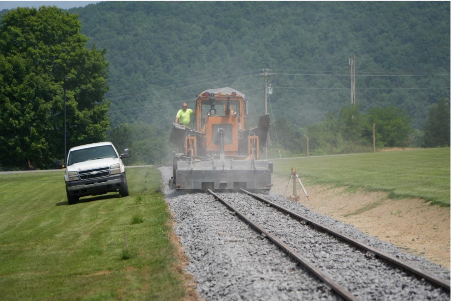
EBTF track foreman Henry Long smooths FEBT campaign-funded ballast in front of the high school. – Al Gallo photo
