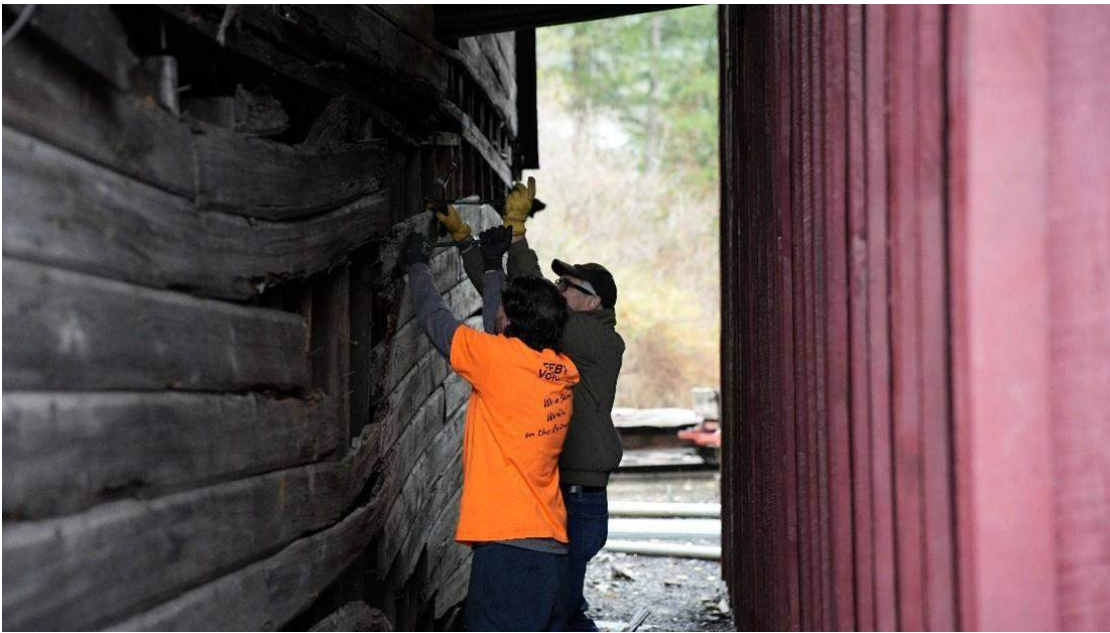
Stephen Ramirez and Dave Bulman remove deteriorated siding on Storehouse 2. — Jacob Bury photo
