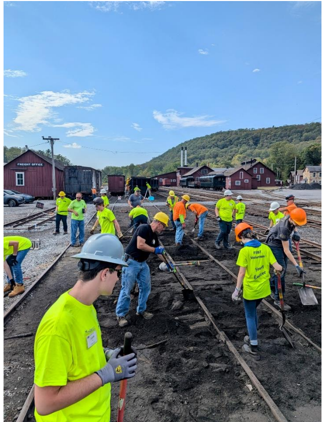
Young Easties work on replacing ties in the Rockhill Yard during the September 2024 session. – Justin Santichen photo
