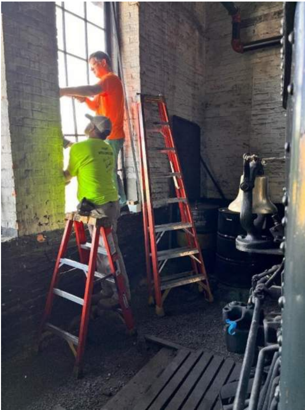
Left: The Glass Rattlers installing the final restored sash in the roundhouse. – Dave Bulman photo
