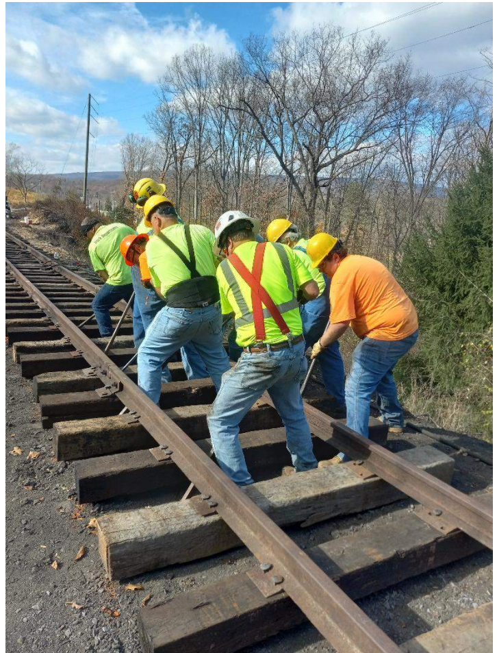
Track crew members align main line rail on the south face of Jordan Summit in November 2024. – Gene Tucker photo
