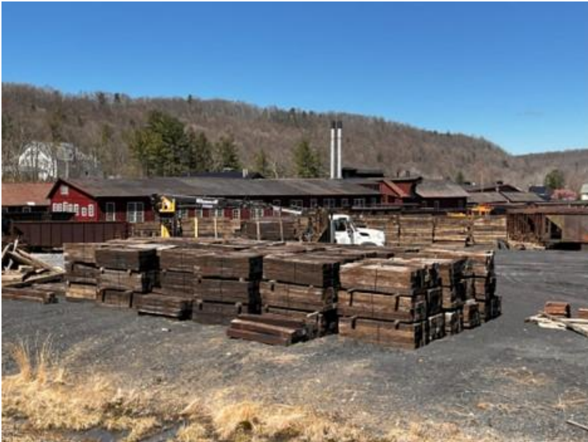
A huge quantity of ties staged in the Rockhill Yard all funded by the FEBT Campaign to support the March to Saltillo. Dave Bulman photo.
