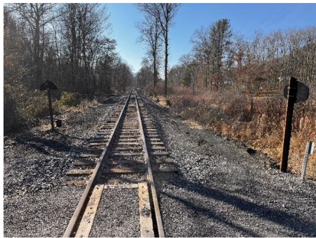
Newly completed track south of IOOF crossing
