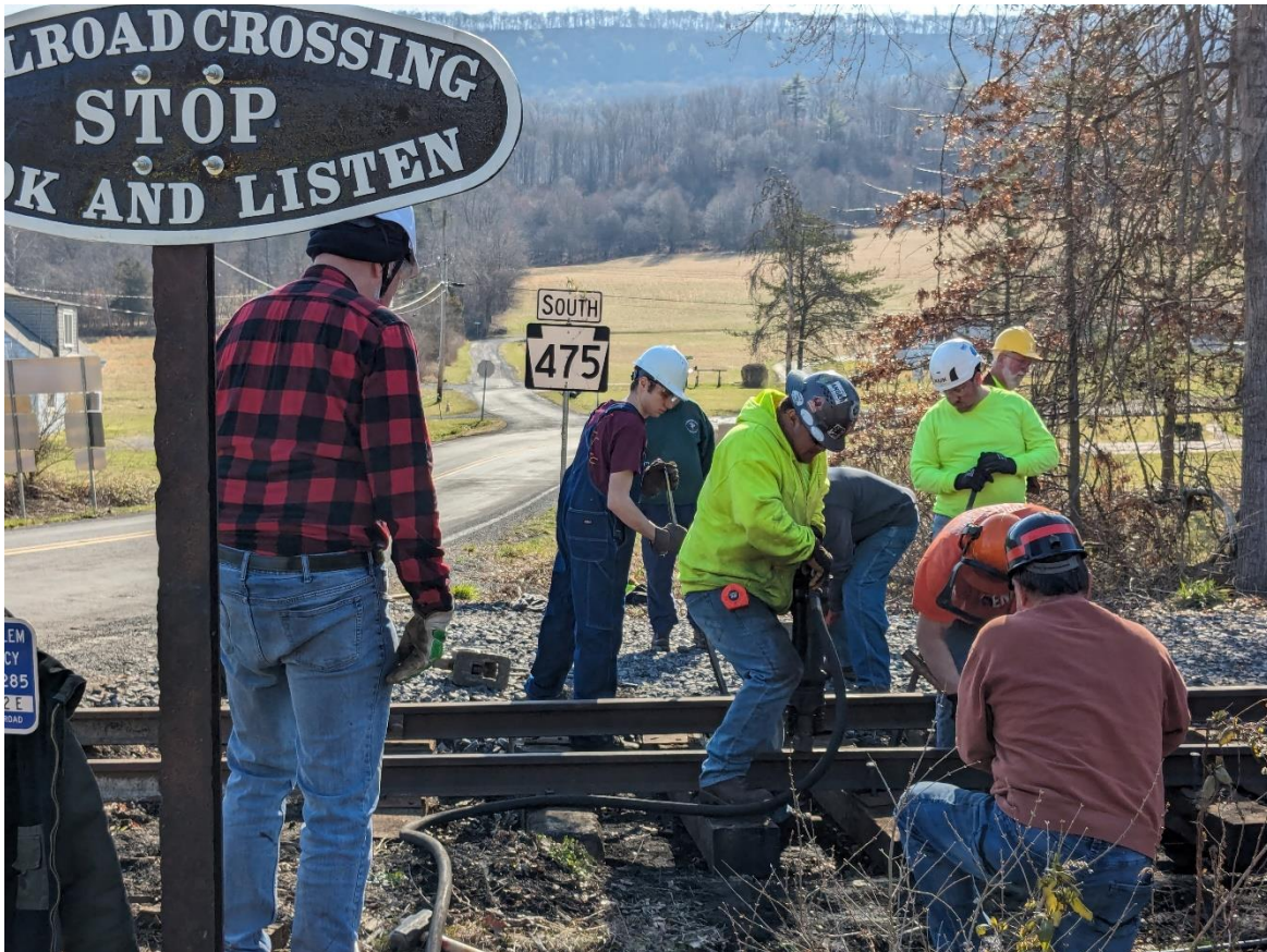
The first few spikes are driven into fresh ties in the Jordan Summit segment of the March to Saltillo. – Al Gallo photo
