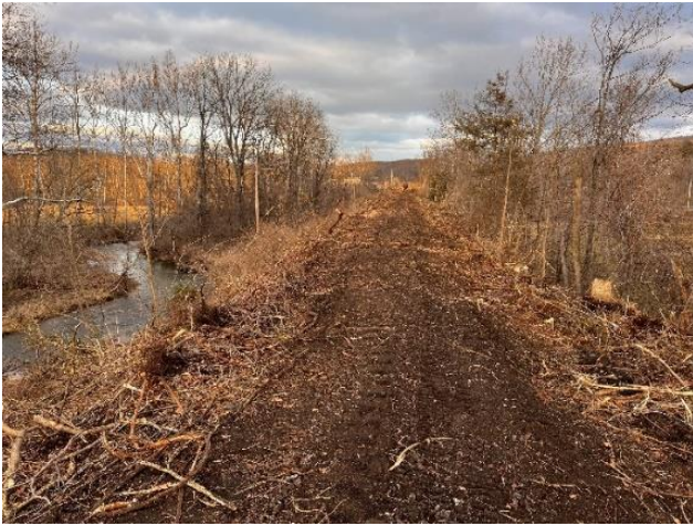
Freshly cleared ROW at Pogue Station
