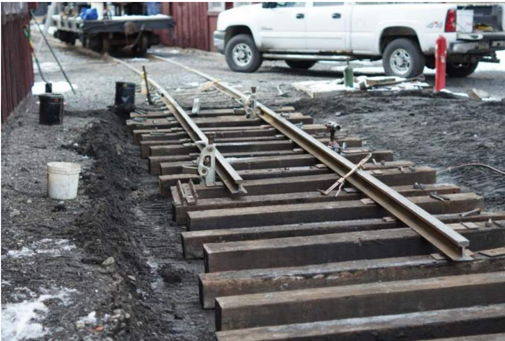
An in-progress view of the trackwork around the inspection pit fill. – Al Gallo photo
