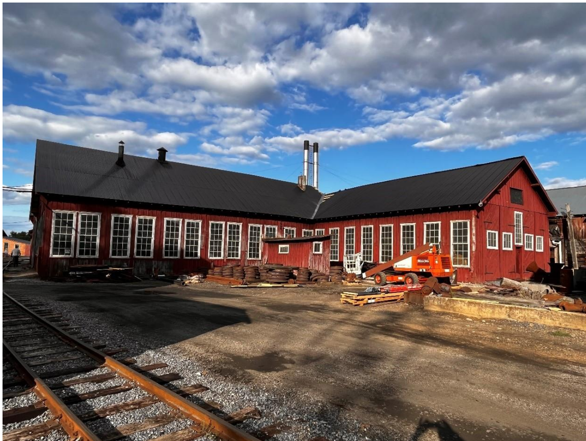
Above: FEBT's work crew installs a new coupler during a summer 2023 work session. – Dave Bulman photo
