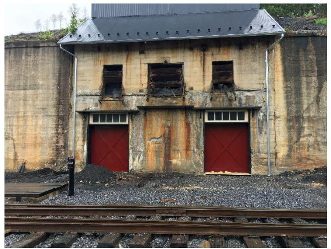
Before and after photos of the new coal dock doors, transom windows, gutters, downspouts, and above-door platforms constructed by Brad Esposito, James Roslund, Kari Roslund, and Craig Confair during the FEBT Fall Work Week. – Left photo on September 18 th by Craig Confair, right on September 23 rd by Brad Esposito
