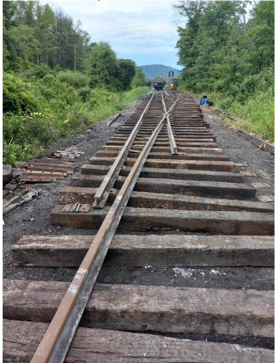
A northward view from the Oddfellows Cemetery Road grade crossing. The Coal Dock Filling Shed is visible in the distance, over a football field away. The extent of tamped ballast in the main line is in closer proximity to the switch at the southern-most point of the Rockhill Yard. – Gene Tucker photo
