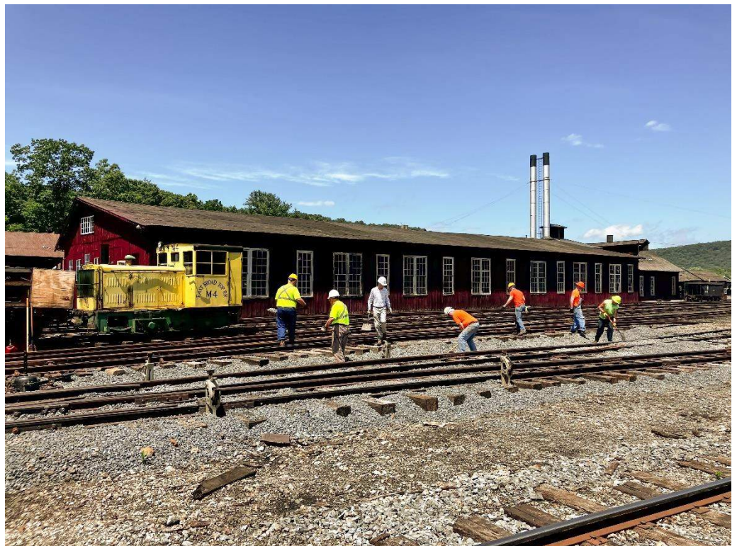
Below: Track crew members manually regulate ballast around the switches at the south end of the Rockhill Yard. – Eric Knepp photo
