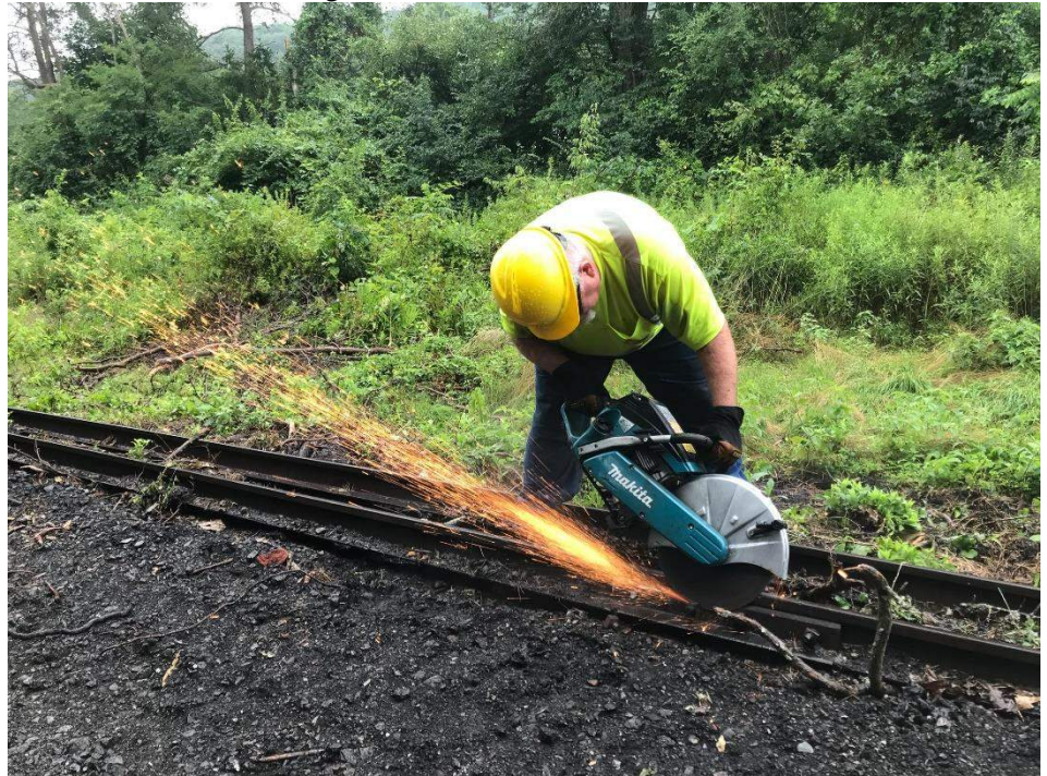
Dave Hart cuts bolts in the rails on the north face of Jordan Summit during the late July work session, as the March to Saltillo makes its way up the grade. – Tim Schindele photo
