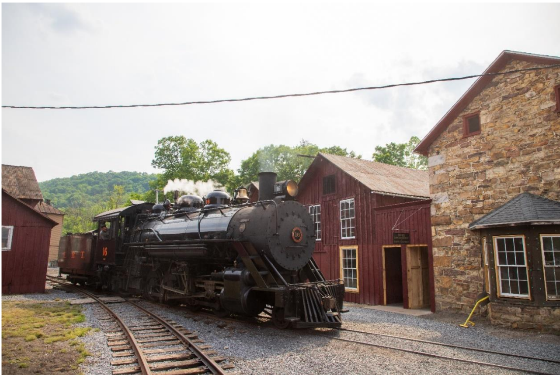
No. 16 returns to the Rockhill roundhouse, passing the nearly-completed Storehouse lean-to project. – Eric Knepp photo
