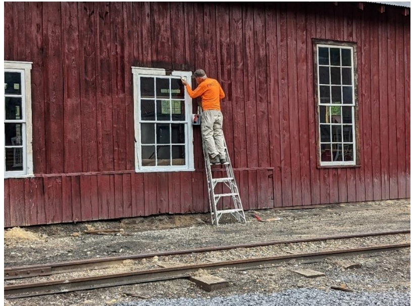
Al Modro paints the trim around a freshly installed window sash in the west wall of the Car Shop. – Al Gallo photo
