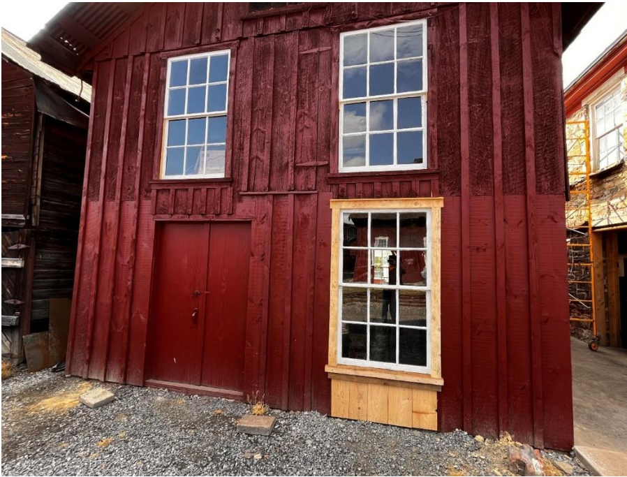
The completed Storehouse first floor window. The sill of this window was below ground prior to the Storehouse restoration. The opening had been used as a temporary door to move hardware back into the first floor. – Dave Bulman photo
