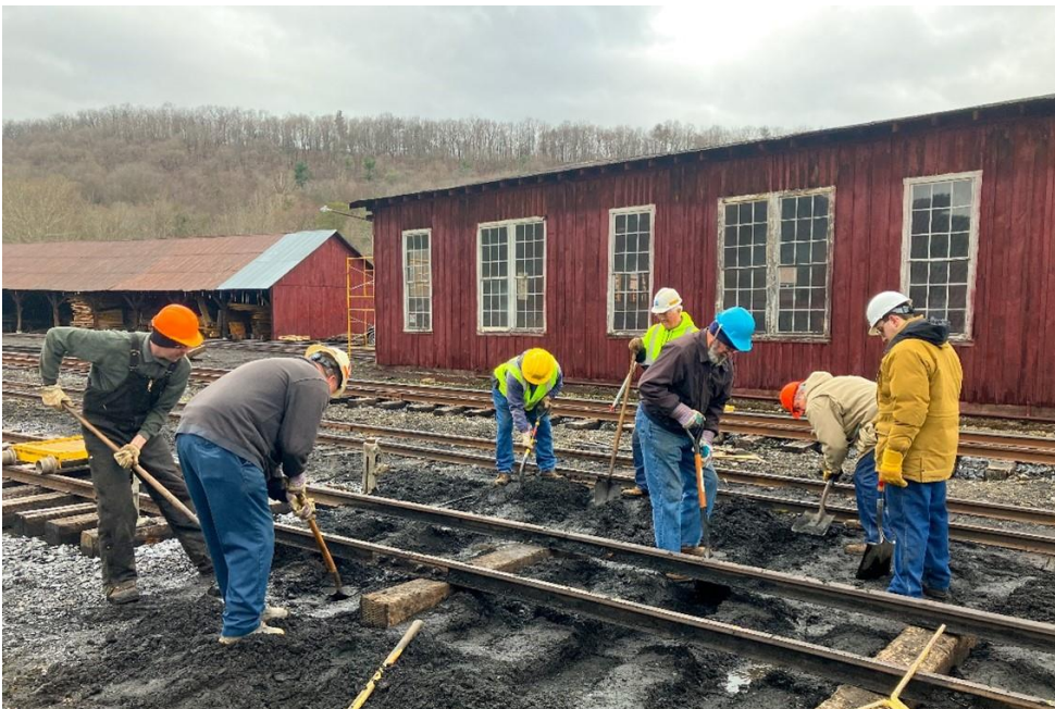
FEBT Track Crew members Derick Erwin, Tom Perman, Gene Tucker, Larry Fuchs, Mark Reese, David Syiek, and Greg Syiek dig cribs to insert ties under the rails of Track 4 alongside the Car Shop during the March 2023 Work Session. – Eric Knepp photo
