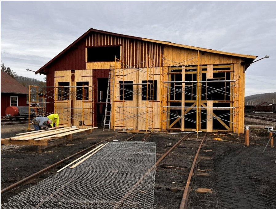
Tom Perman and Craig Confair prepare siding boards for installation on the Car Shop doors during the February Works Session. – Dave Bulman photo
