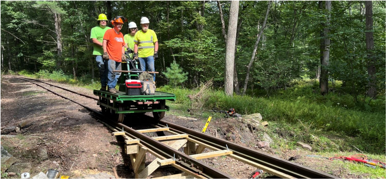
FEBT Track Crew members test their work with a handcar ride over the new trestle. – Todd Johnson photo
