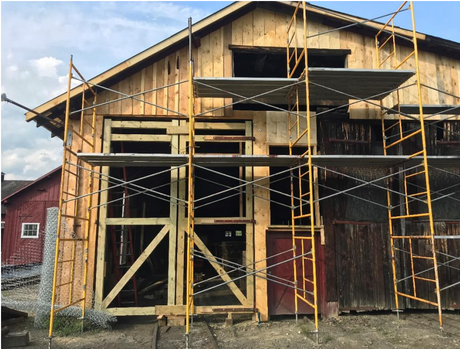
The south end of the Car Shop, at the conclusion of the September Work Session. Lots of replaced boards are clearly visible. – Crag Confair photo
