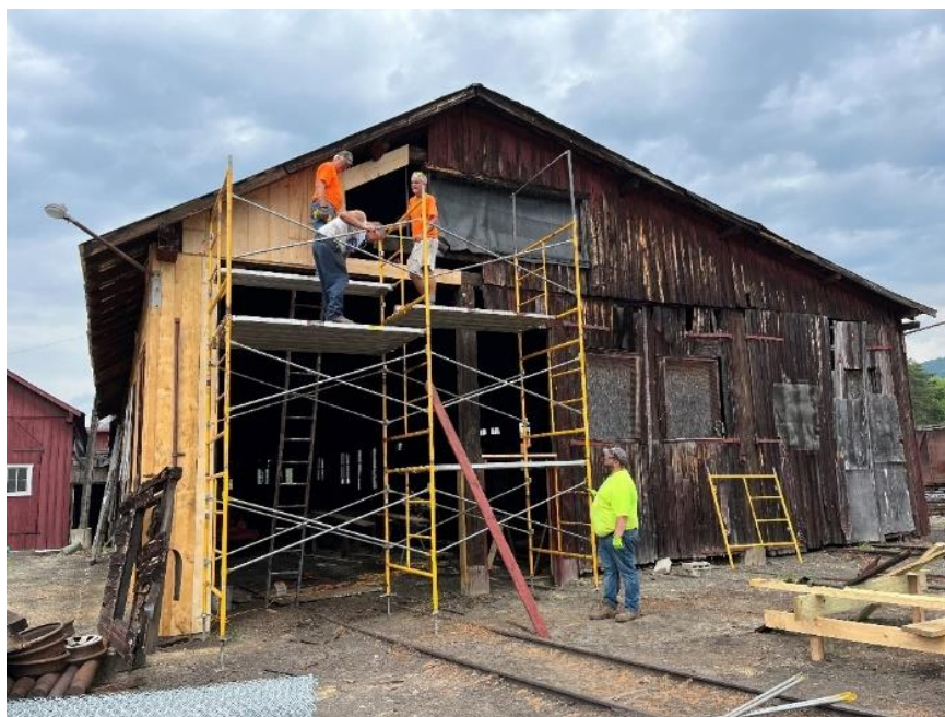
FEBT members Larry Fuchs, Tom Perman, Craig Confair, and Joel Myers perform some sorely needed carpentry work replacing wooden sheathing on the south end of the Car Shop in the Rockhill Shops Complex during the July 2022 work session. – Dave Bulman photo
