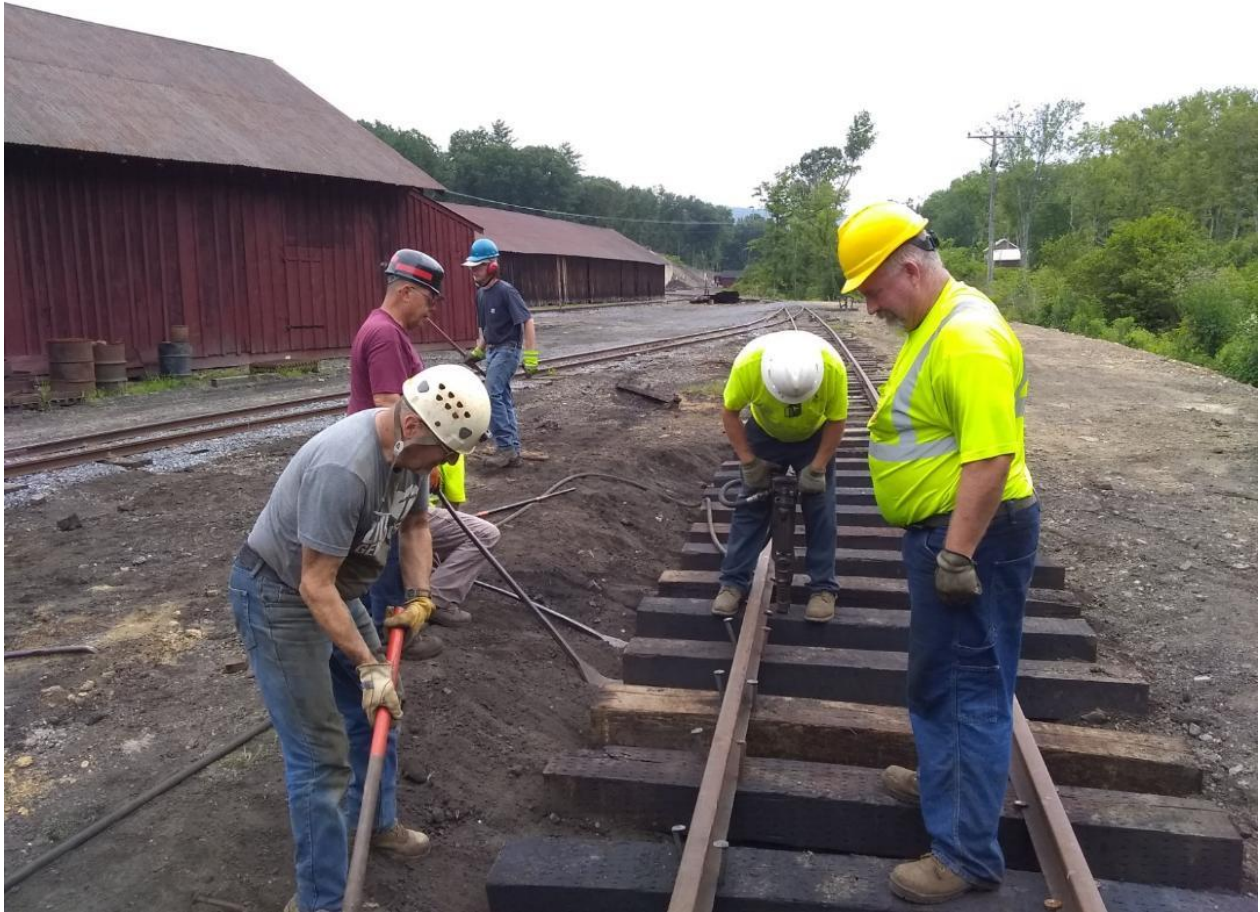
The FEBT Track Crew works together to spike up the Paint Shop lead track during the July work session. – Larry Fuchs photo
