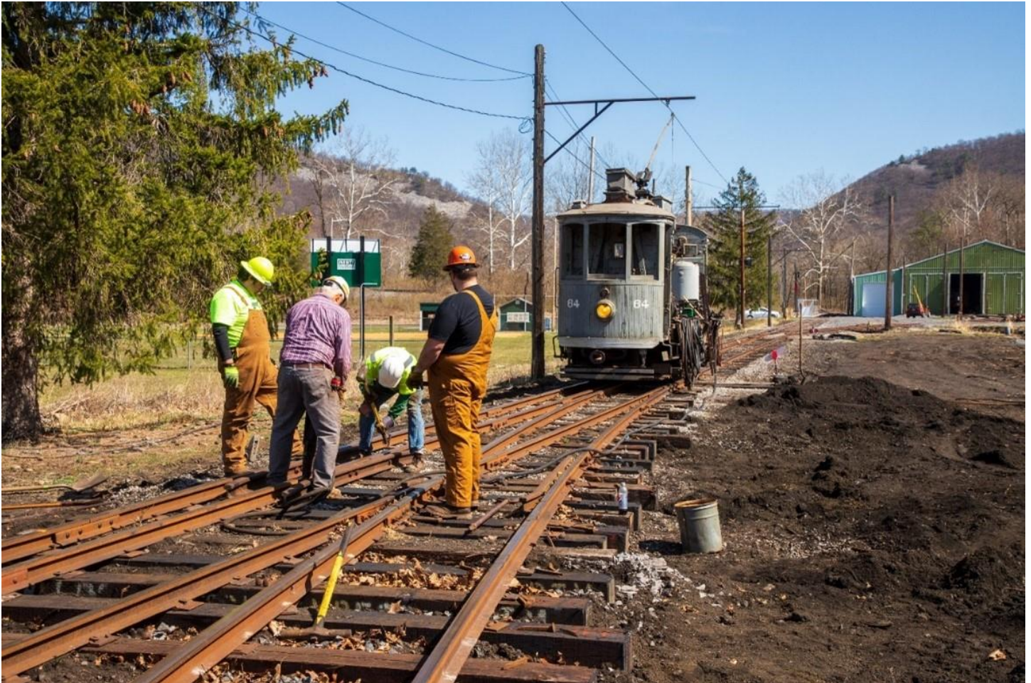
Track crew members Kevin Conklin, John Quinn, Larry Fuchs, and Justin Santichen work on switch repairs on the dual gauge Rockhill Trolley Museum trackage that is part of the east leg of the Rockhill wye. Car C-64 is RTM's work car, built in 1905. – Eric Knepp photo.
