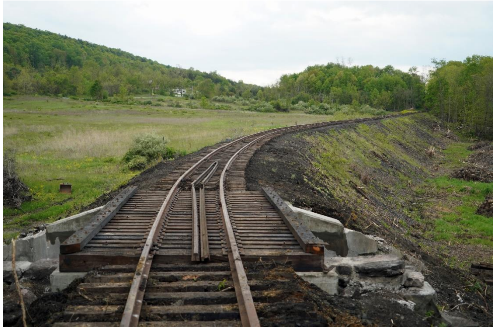
A southbound view of the restored trackage across the Runk Road bridge and long fill on May 11, 2021. Ballast work would be completed over the following 10 days. – Craig Confair photo
