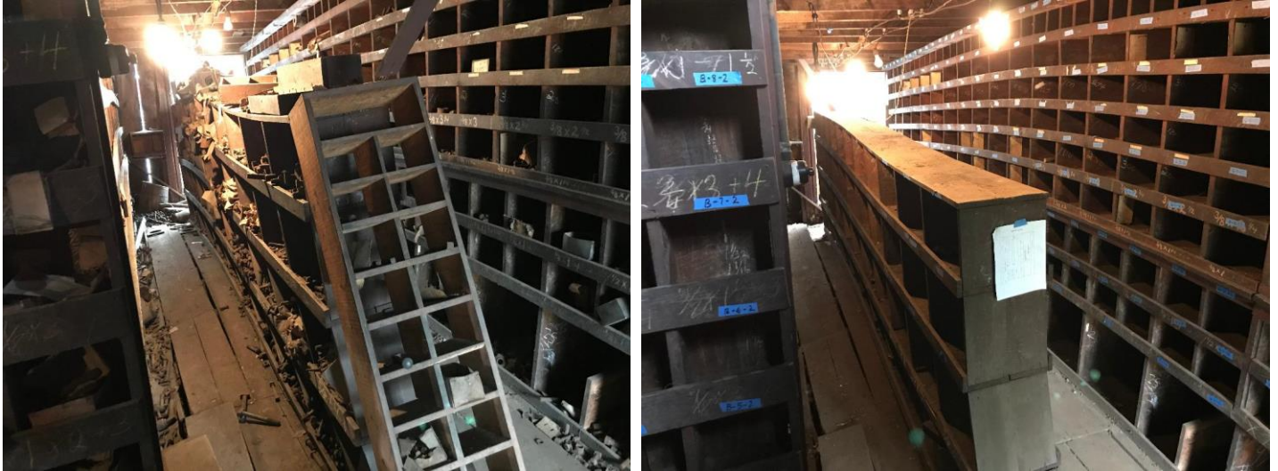
Before and after photos of bins withing the Storehouse. It is not an optical illusion that the bins are bowed, it is a sign of how much the building has sunken over time, and why this project is necessary. – Dave Bulman photos
