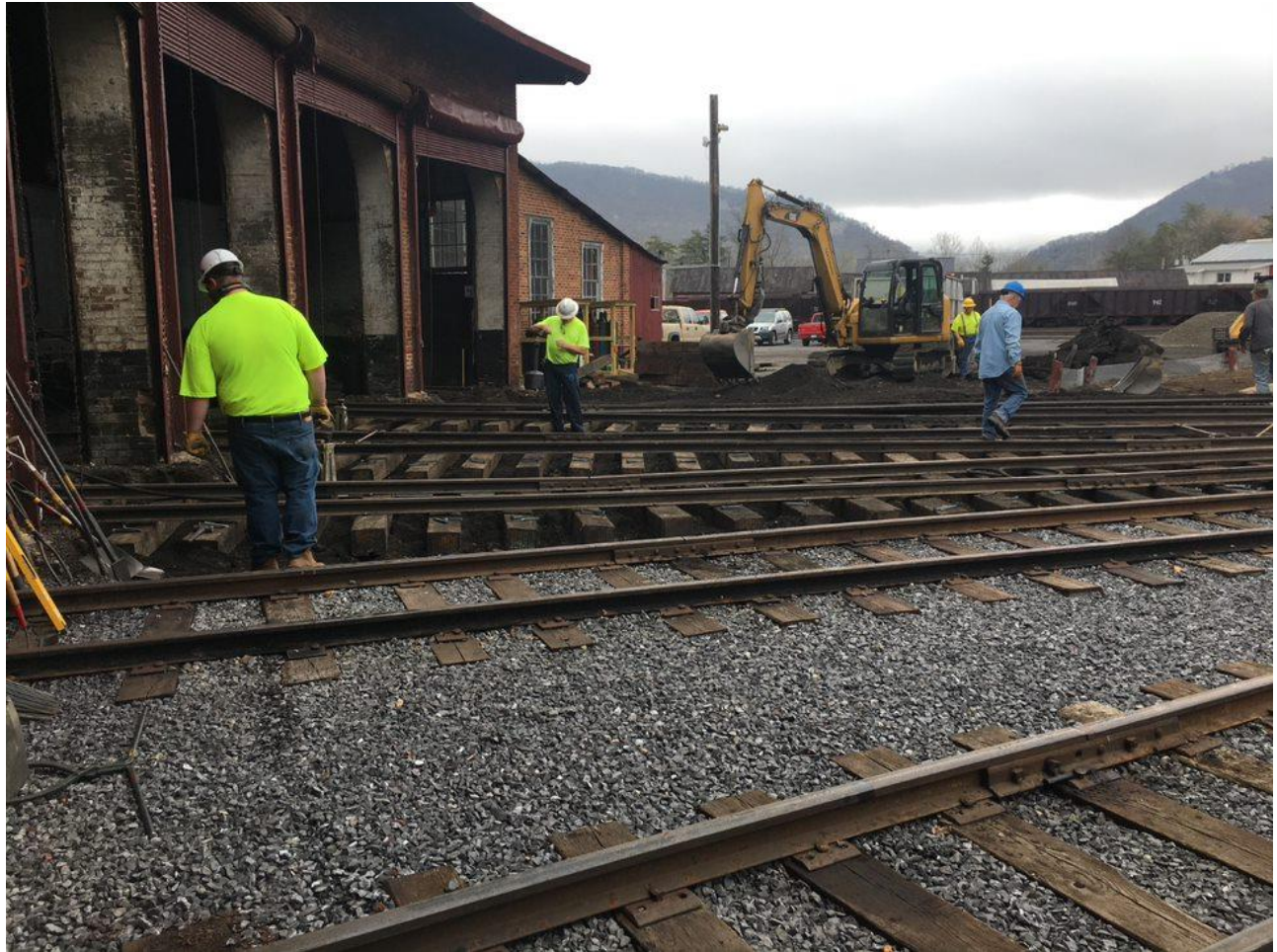
FEBT Track Crew rebuilds the roundhouse leads to the eastern half of the stalls during the April work session – Todd Johnson photo
