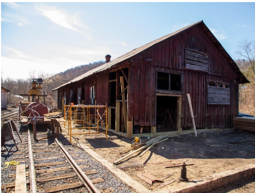
The Carpentery Shop sits stabilized and awaiting new board and batten cladding on March 13, 2021. The stabilization was an FEBT-funded project, and the remaining restoration work will be performed by FEBT members during work sessions. – Eric Knepp photo
