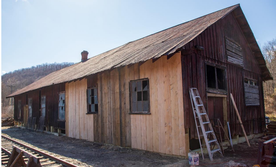
Top: The Carpentry Shop leans in disrepair in the fall of 2020. – Brad Esposito photo Bottom: FEBT members installed new board siding during the March 2021 work session, after the stabilization had been completed. – Eric Knepp photo
