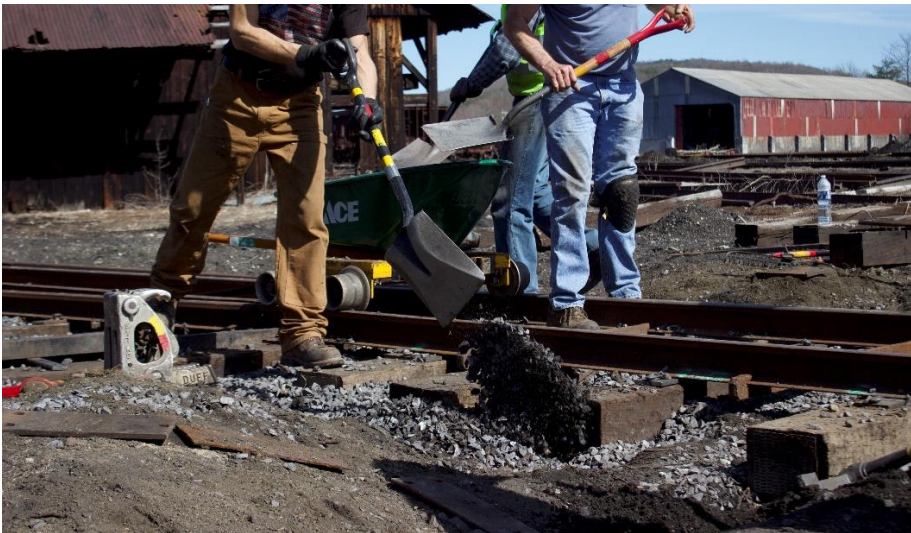
FEBT track crew members fill the cribs between recently replaced ties with ballast on the ladder track during the March work session. – Wayne Wanzor photo
